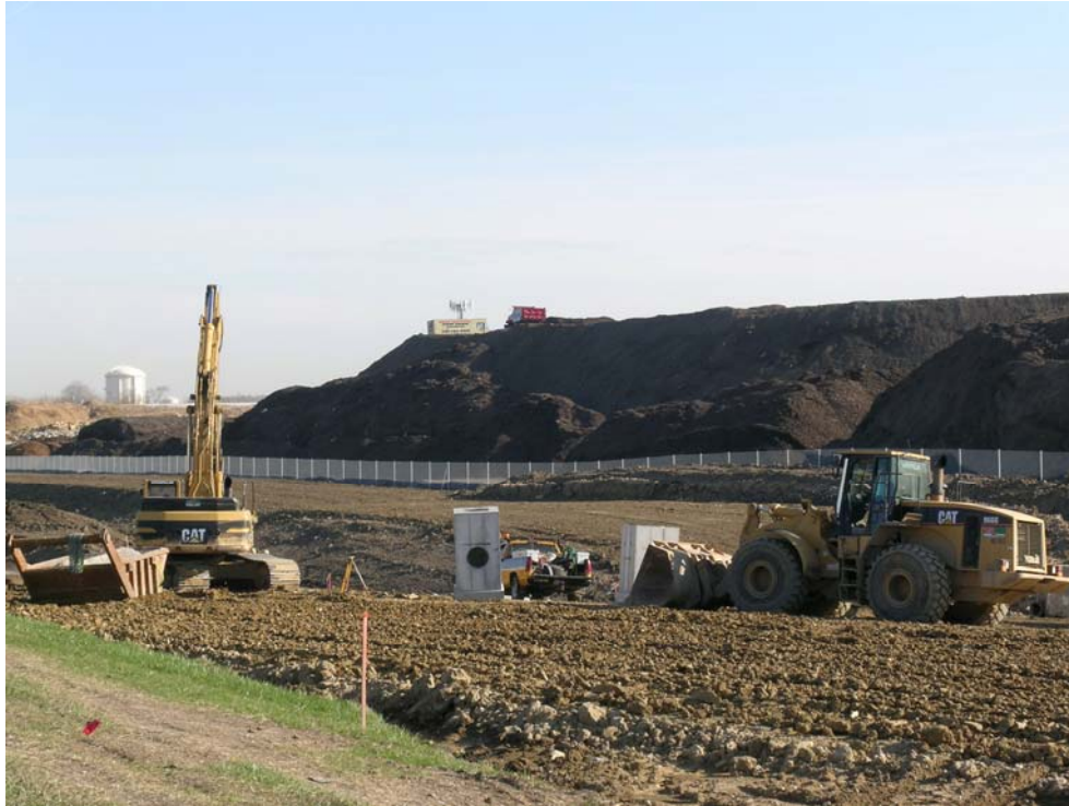
Grading work continues at the I-355/I-55 interchange.
